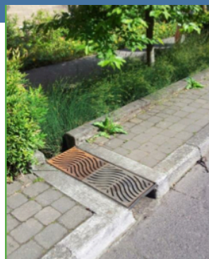
Trench drain and rain water scuppers at terrace wall for bioswale
